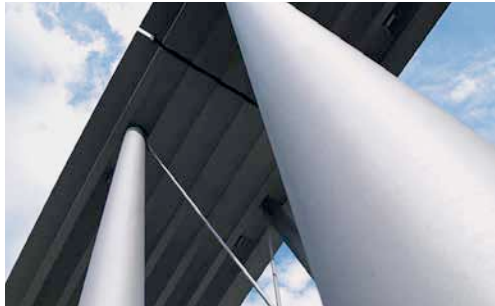
Bridge construction with textile reinforcement
